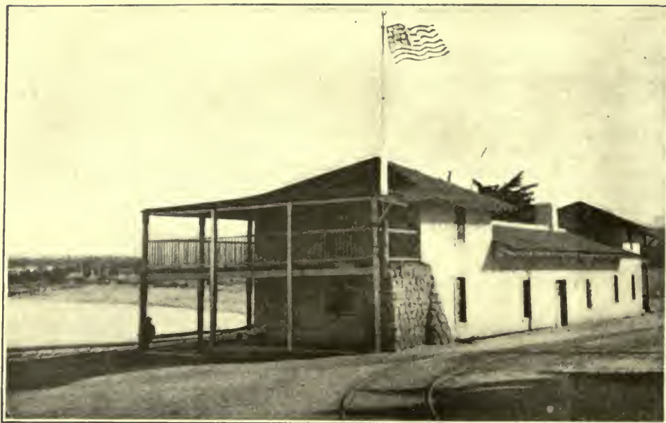
WHERE COMMODORE SLOAT FIRST RAISED THE AMERICAN FLAG OVER CALIFORNIA—Old Custom House at Monterey where the Constitution of California was formulated and the Stars and Stripes proclaimed it to the world as the Golden Gate to the American Republic as related in Captain Aram's journal
